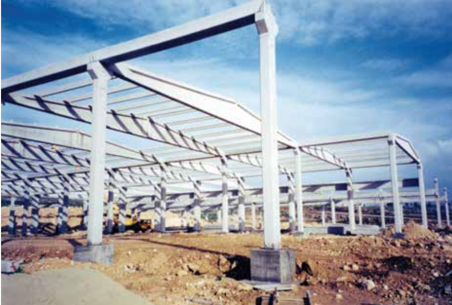
The beginnings of the new plant
